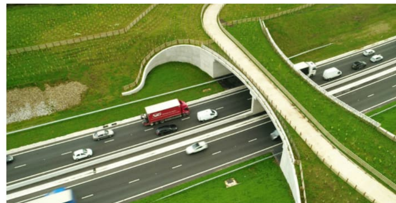
Figure 14: Photograph of an existing green bridge on A556, west of Mere (photograph courtesy of National Highways)
