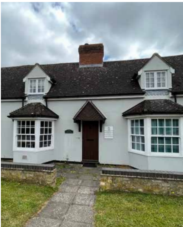
Figure 74: Porch, sash, bay windows and dormers
