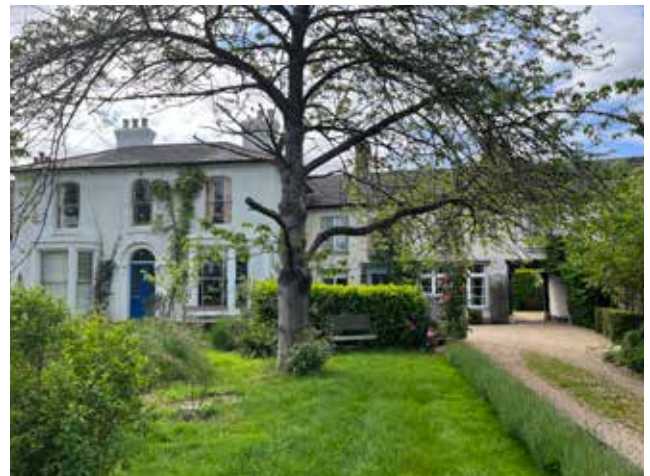
Figure 23: Semi-detached 2 storey buildings with deep front gardens
