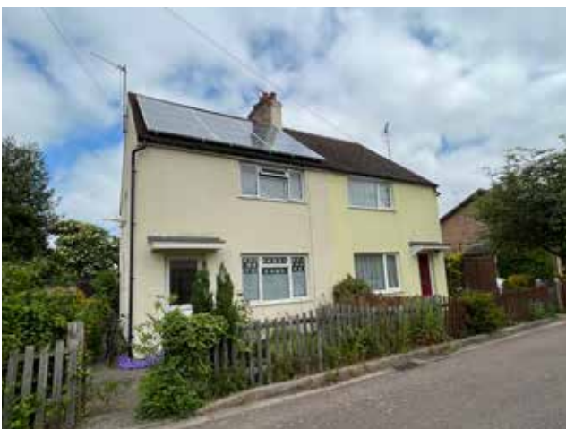
Figure 62: 2 storey semi-detached houses with narrow front garden
