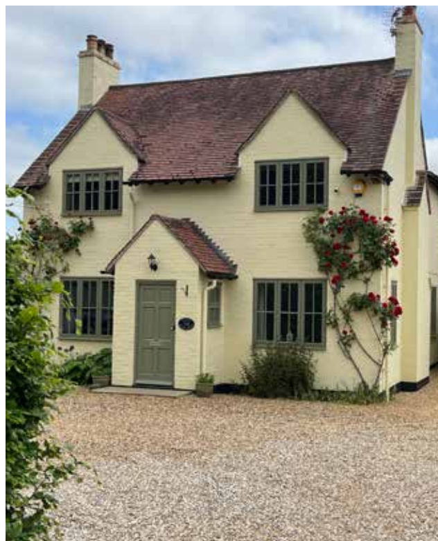
Figure 70: Well proportioned sash windows and centred protruded porch painted in olive green on a cream painted brick frontage
