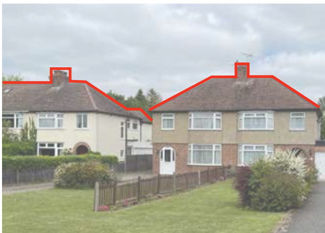
Figure 68: Example of hipped roofs along London Road
