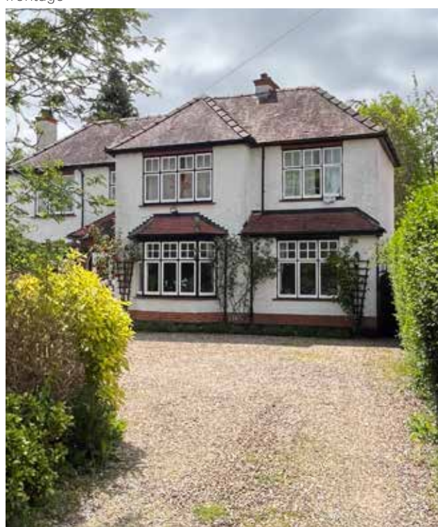
Figure 71: Mix of casement and sash windows with a bay window at the ground floor.
