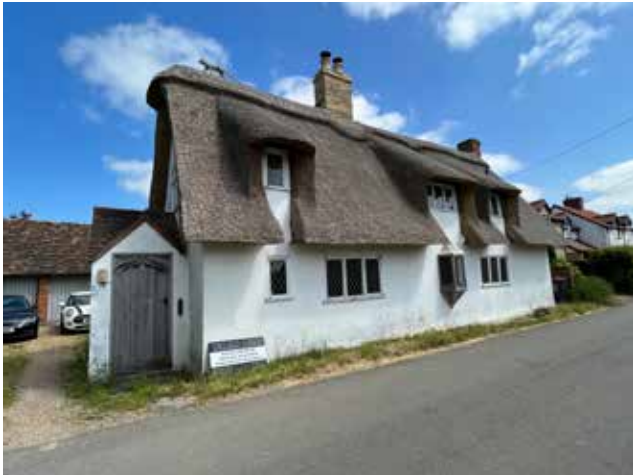
Figure 13: Hope Cottage, 2 storeys with thatched roof
