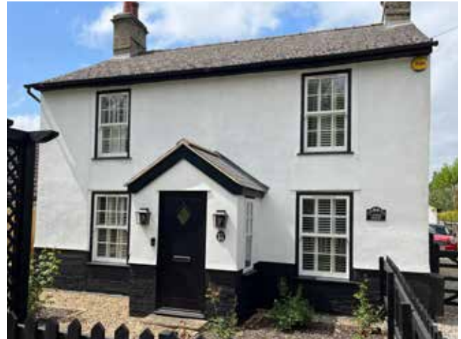
Figure 40: Detached house with white render facade and decorative basement fascia in brick painted black
