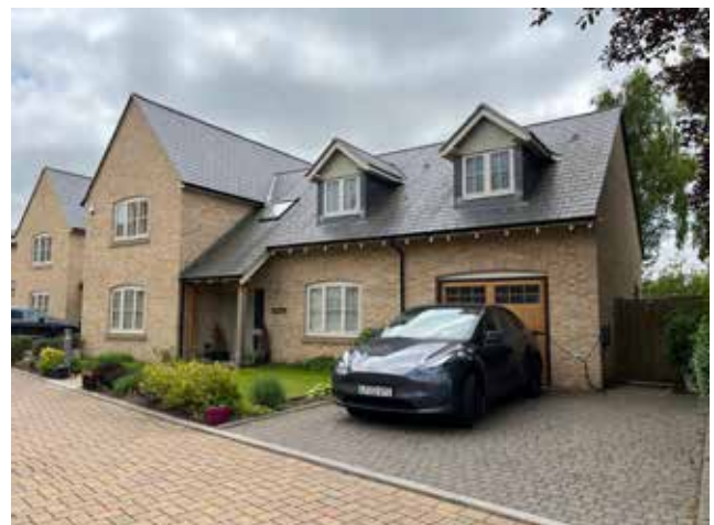
Figure 60: The Pastures. New development using traditional materials
