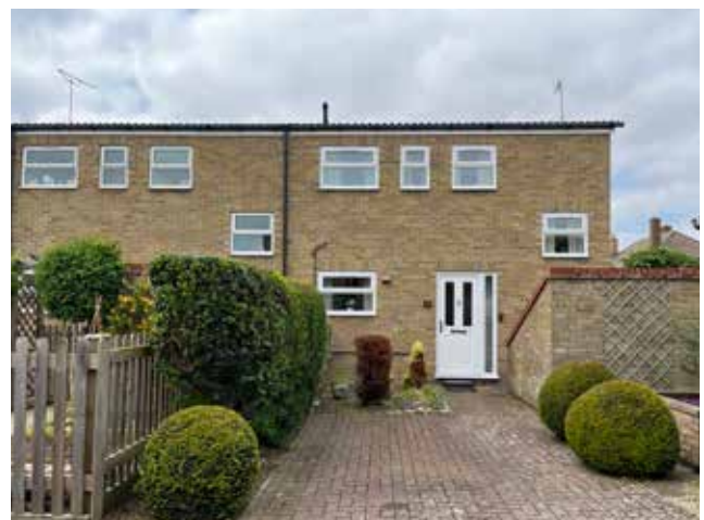
Figure 65: 2 storey semi-detached houses with buff brick
