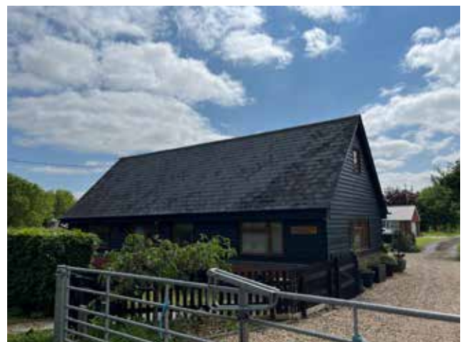
Figure 17: Parkfield converted commercial building
