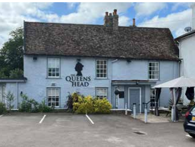
Figure 21: The Queens Head, local restaurant. 2 storeys building with sash windows and a slated roof
