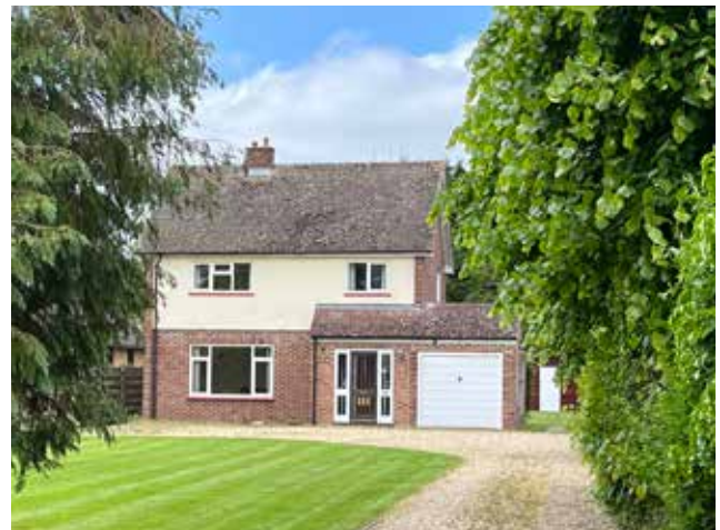
Figure 48: Detached house with pitched roof
