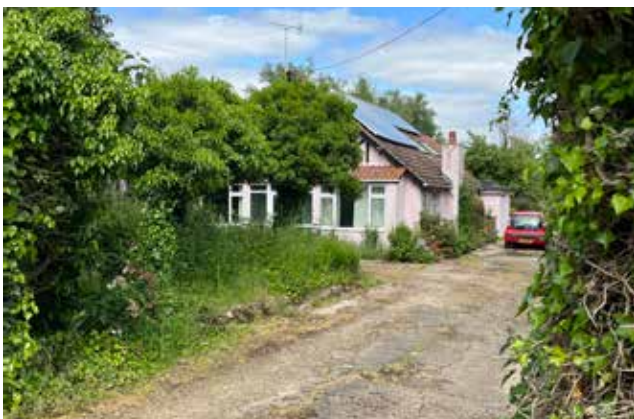
Figure 91: Large landscaped garden with tall hedgerows and trees that conceal the building in CA1.
